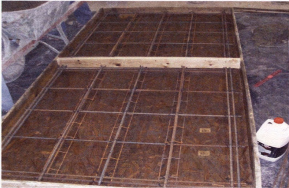
Figure 3.5 – Reinforcing Steel Layout in Forms
