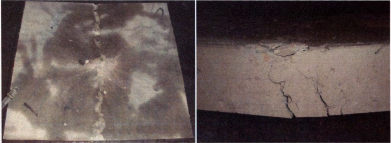
(a) Concrete Crushing on Compression Face (b) Flexural Cracks on Front Face
