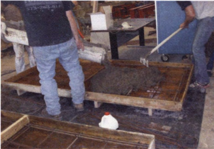
(a) Pouring of SFRC
