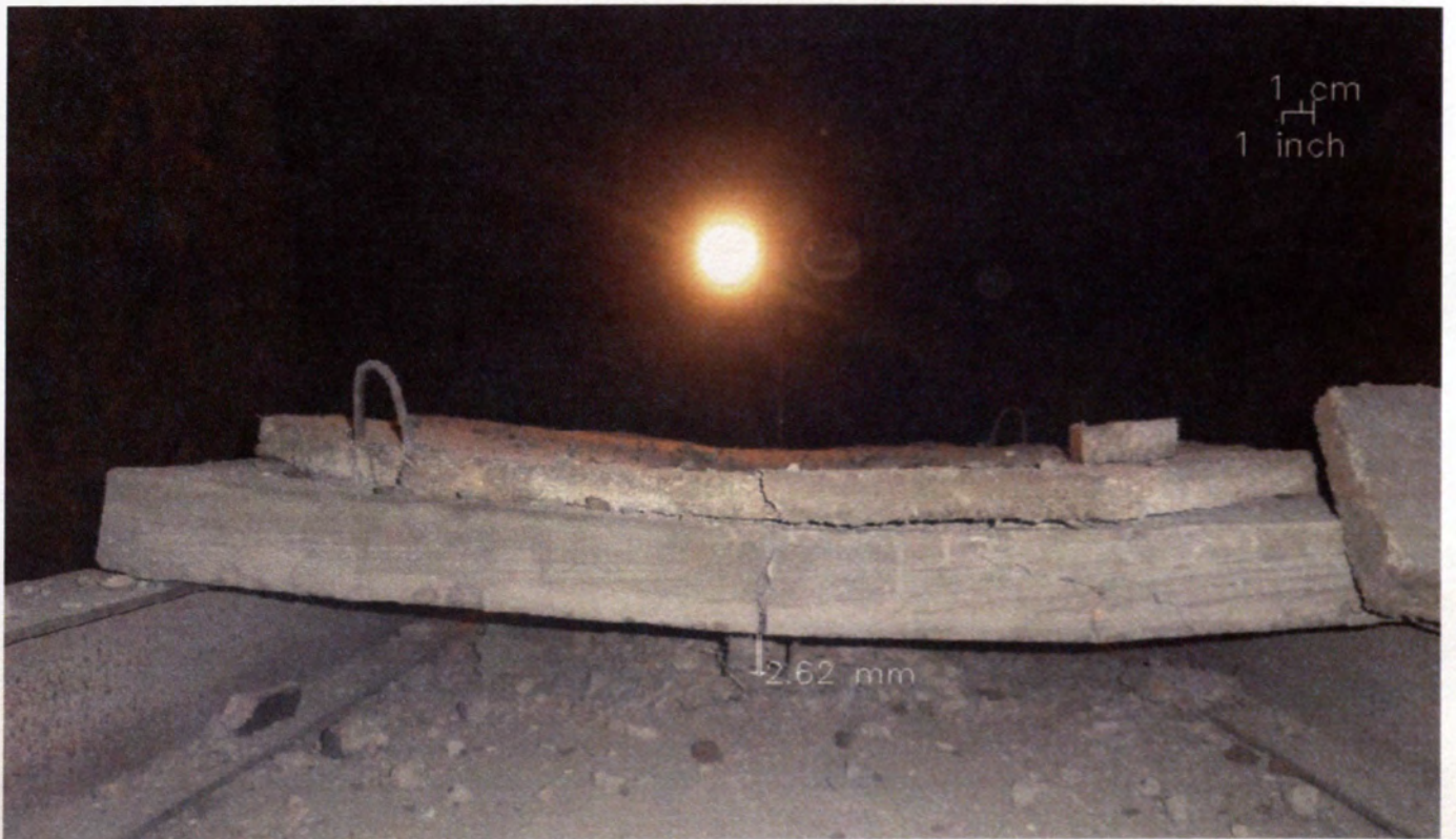
Figure E.9 – Flexural Cracks in the Back Face of 2-H, 2 nd Event
