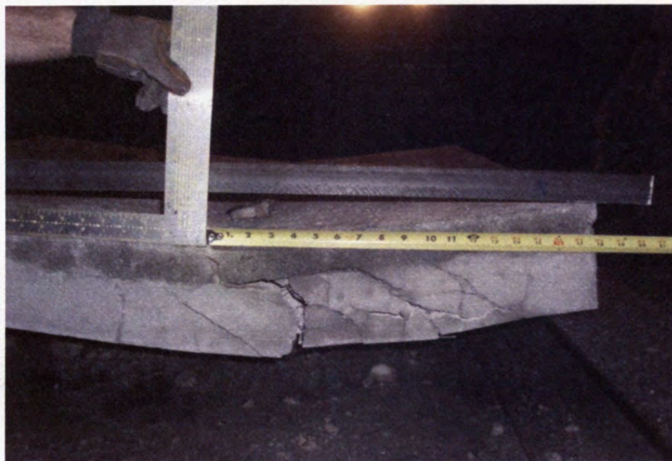
Figure 3.12 – Measuring Residual Deflections
