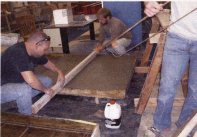
(c) Leveling with Screed
