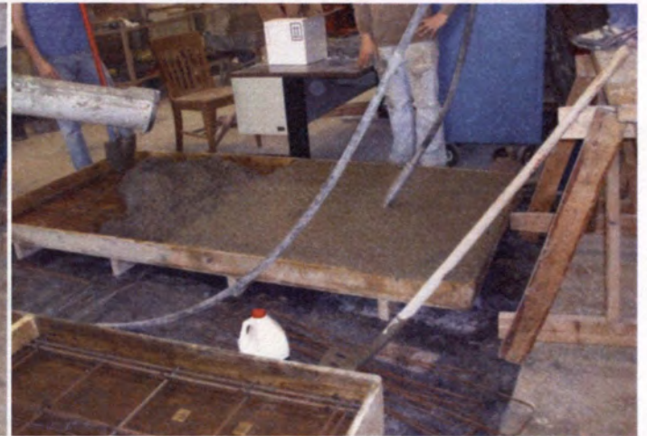
(b) Vibrating the Concrete
