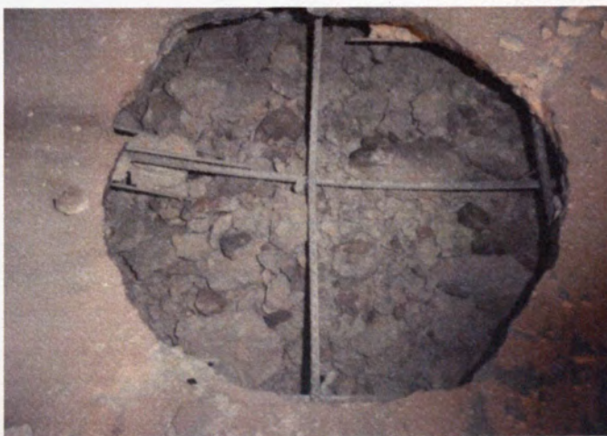
(e) Hole From Above the Panel
